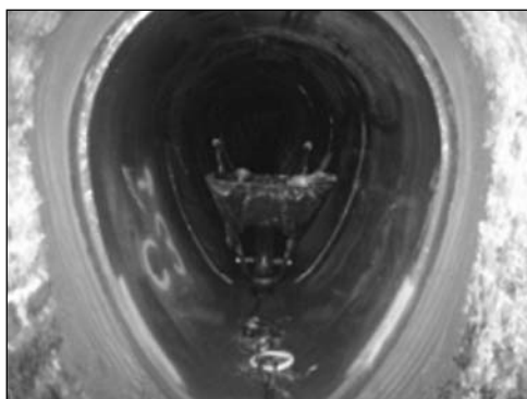
Figure A3.31 Installation of GRP pipe and grouting between annulus around GRP pipeline and behind timber heading
