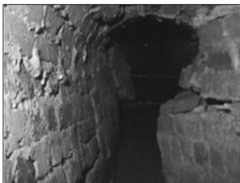
Figure A3.26 Inside the barrel of the culvert showing erosion to brick work and lateral movement of the RHS wall
