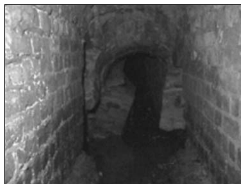
Figure A3.27 View showing lateral movement of sidewalls and partial collapse of roof element
