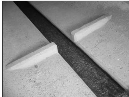
Note the use of a low-flow channel in the centre of the channel.
