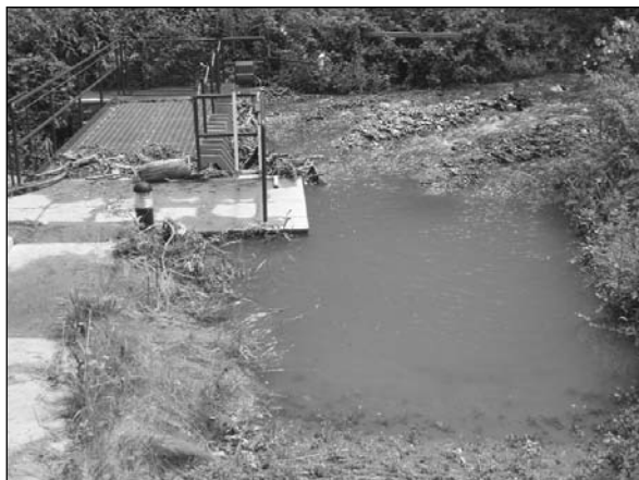
Figure A3.41 River Jordan debris screen following high-flow event in June 2007. Note that debris has accumulated upstream of the screen up to the level of the cleaning platform (courtesy Environment Agency)
