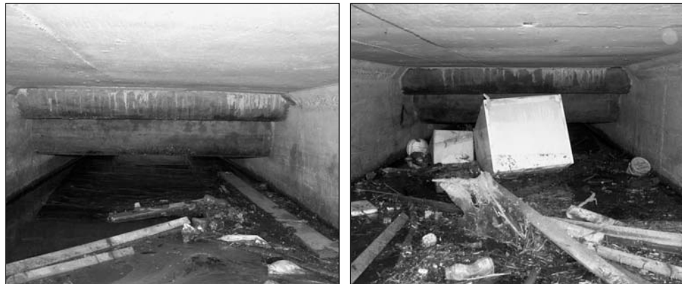
Two service pipes cross this culvert, significantly reducing its capacity and increasing the risk of blockage. Complete blockage could easily occur in a flood, causing severe flooding to local properties and infrastructure. Such blockages are difficult to remove and can only be cleared after the flood event. In the case of an existing situation such as this, the only solution may be to introduce a trash screen at the inlet, but it should be appreciated that this will impose a requirement for routine and emergency cleaning.
