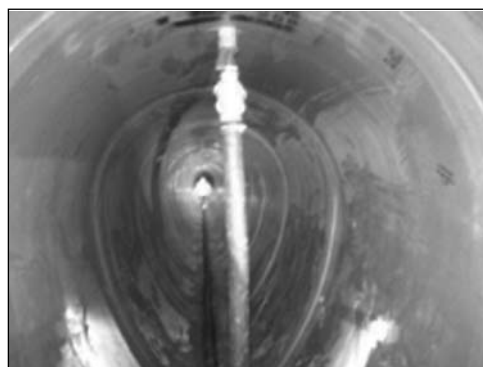
Figure A3.32 View showing completed re-lined culvert
