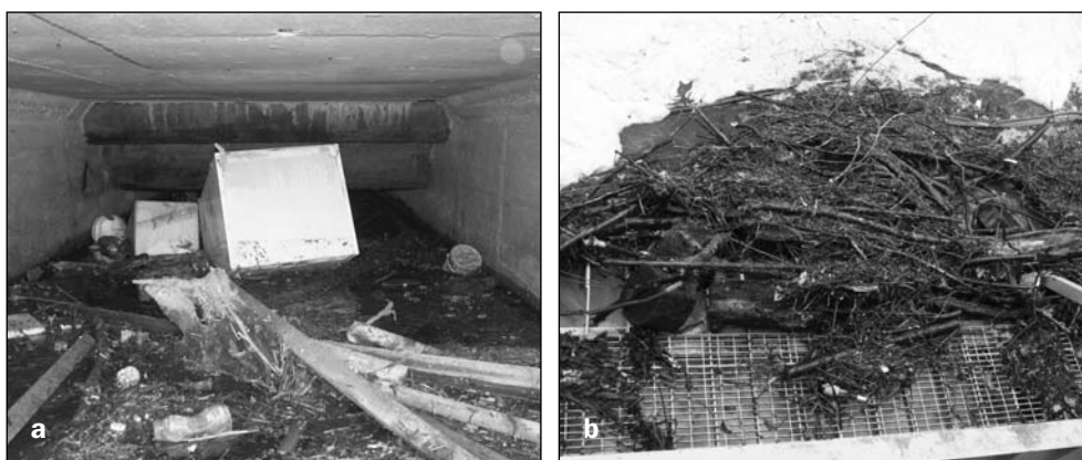
Figure 8.3 Obstructions within a culvert (a) and debris blocking a culvert entrance (b) (courtesy Richard Allitt and Scott Arthur)
