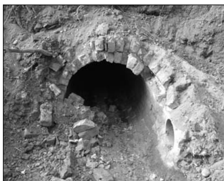
Figure 8.12 The culvert during demolition (courtesy Andy Pepper)
