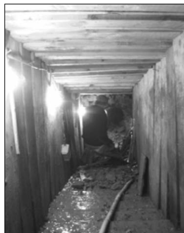
Figure A3.29 Installation of new timber-framed heading
