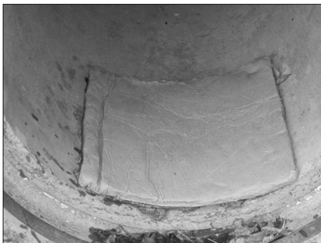
Figure A3.14 Detail of clay pad at culvert entrance (courtesy Dorian Latham)
