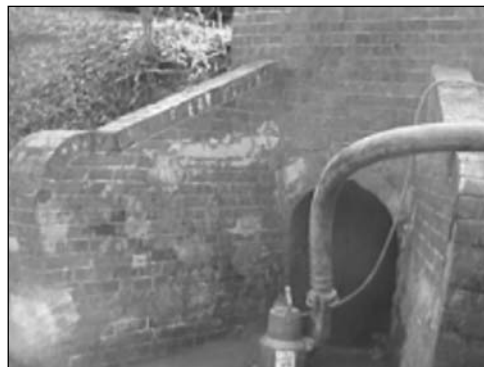
Figure A3.24 Entrance to the culvert, showing large angled brick wingwalls and brick headwall. A pump was used to enable works to be carried out
