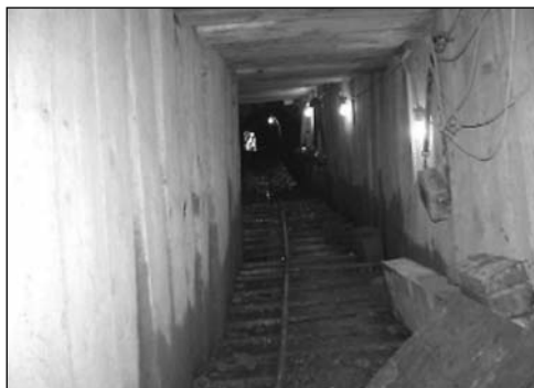
Figure A3.30 View showing completed timber-framed heading
