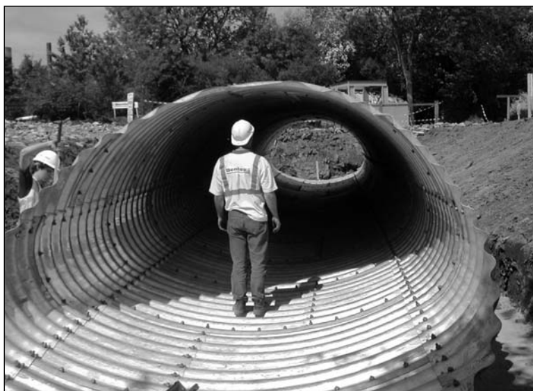
Note how the structure is formed from small panels bolted together on site.
