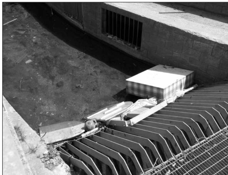
In this case the urban debris has been prevented from entering the culvert by the screen. This type of material could readily block a culvert with severe consequences. Note that there is a bypass facility at this screen to carry flood flows if the main screen is partially blocked by debris.
