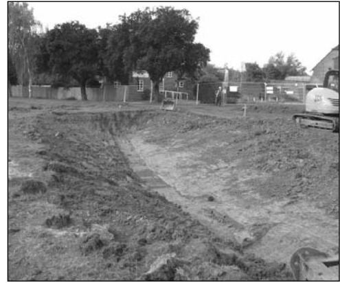
Figure A3.37 Final removal of existing culvert and preparation of new channel bed (courtesy Andy Pepper)
