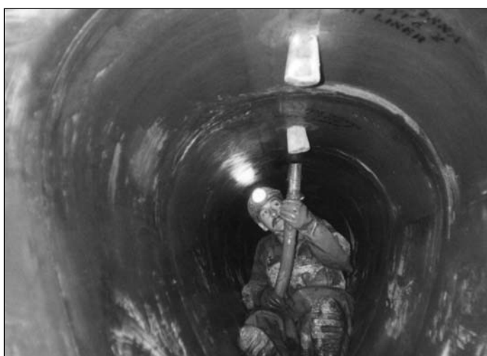
Figure 8.8 Grouting of GRC liner (courtesy Ferro Monk)
