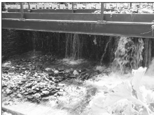
Figure A3.42 River Jordan debris screen following high-flow event in June 2007 (courtesy Environment Agency)
