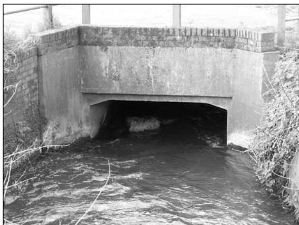
Figure 6.19 Culvert flowing under inlet control
